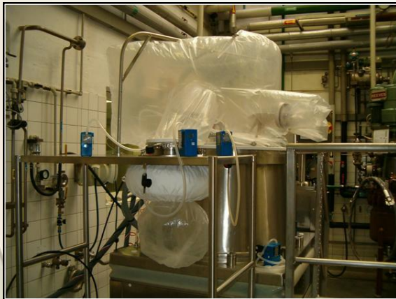
Enclosure and Continuous Liner offload
